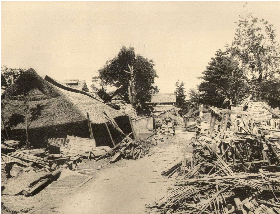
Figure 2. Impact of the 1891 Mino-Owari Earthquake on buildings.: Internet Source
