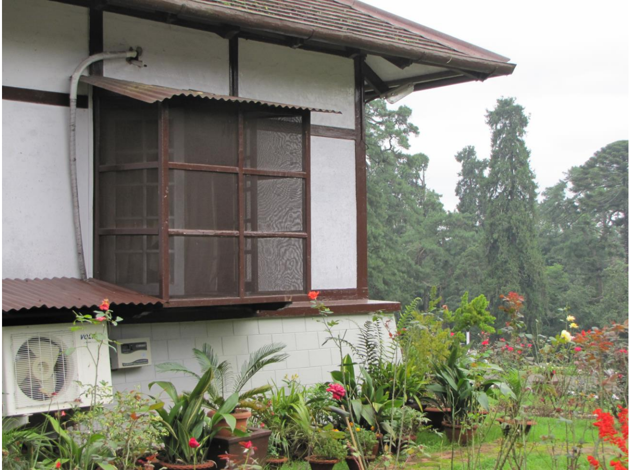
Figure 7. Characteristic features of the 'Assam type' construction after the 1897 Earthquake in Shillong. (Source: Author)
