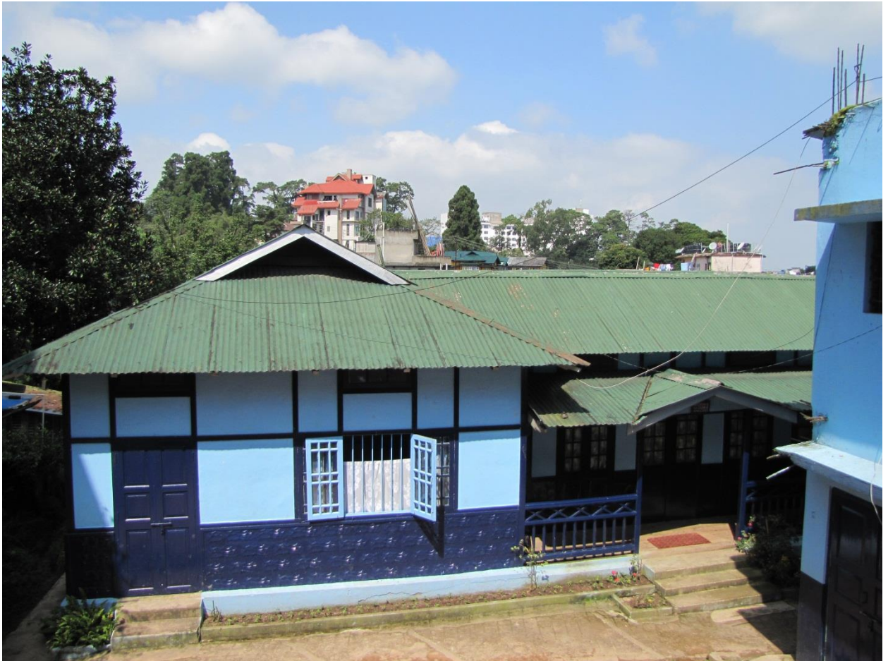
Figure 9. Earthquake resistant ‘Assam type’ construction system after 1897 in the North-east region as heritage resources.(Image: Author, 2015)
