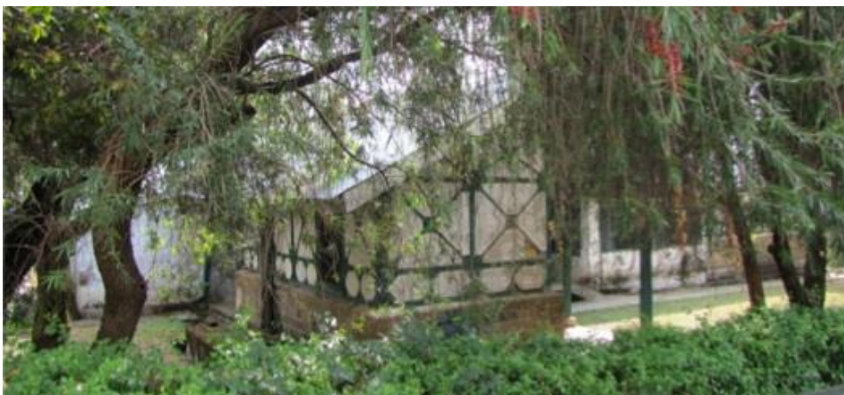
Figure 8. Earthquake resistant construction type after 1905 in the Kangra area (Source: Author)
