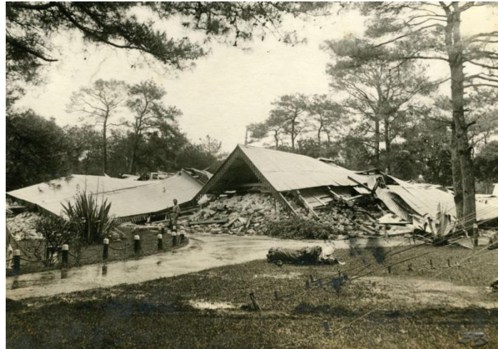
Figure 5. Impact of the 1897 Great Assam Earthquake on buildings in Shillong. Internet Source- Bilham 2008
