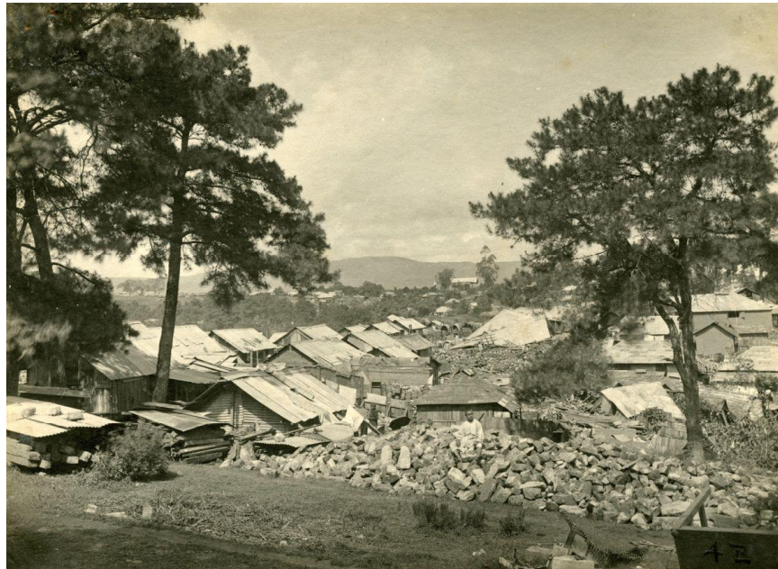
Figure 3. Impact of the 1897 Great Assam Earthquake on buildings in Shillong.: Internet Source C.P.K.Rajendran 2003 and Bilham 2008
